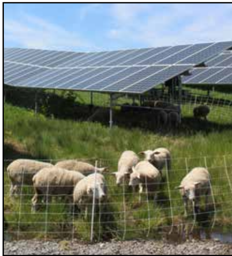
Moveable electro net pen keeps the flock safe while panels provide shade.
